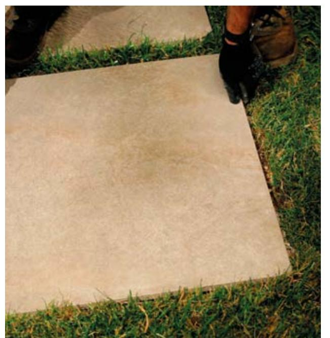
Aextra20 can be easily installed onto grass substrates simply by following the recommendations set out here: trace the encumbrance of the slabs and dig the substrate up to 3 cm. Then apply a layer of gravel to ensure perfect drainage and proceed with the installation of slabs always checking the planarity of the surface.
