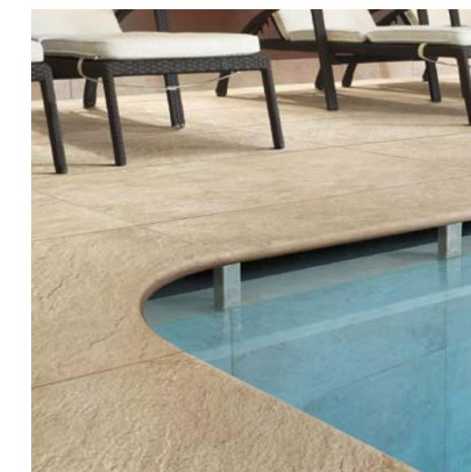
With the internal deck-level solution, the edge of the pool in 20mm thick porcelain stoneware is placed above the draining system, therefore it is concealed and allows for a pleasant "suspended effect".
